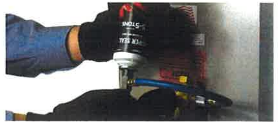
SUPER SEAL ADVANCED™の充填
